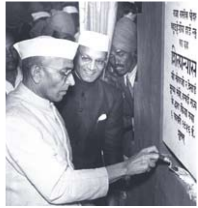
Shri Morarji Desai, Chief Minister of Bombay, laying Foundation of Raja Ramdeo Podar Higher Secondary School. Seen- Dr. Ramnath, Jaipur (1956).
