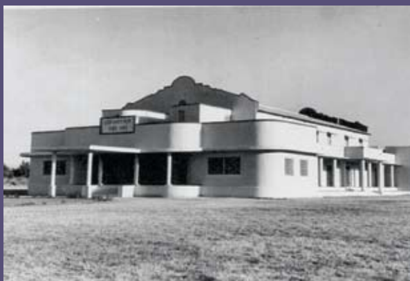
Raja Ramdeo Podar Smriti Bhawan (Cultural Centre) Nawalgarh
